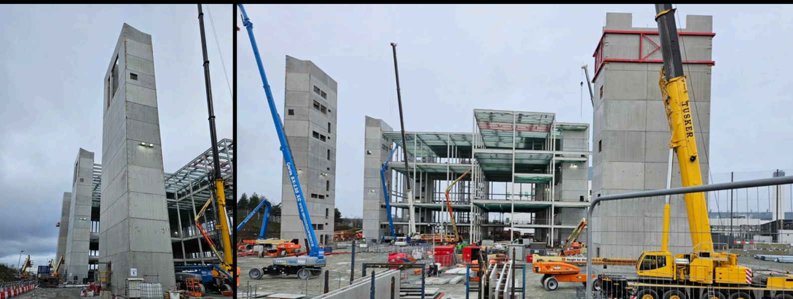
Provided Cranes and lifting solutions to assist Tusker contracts in erection of 8 no. Precast cores
