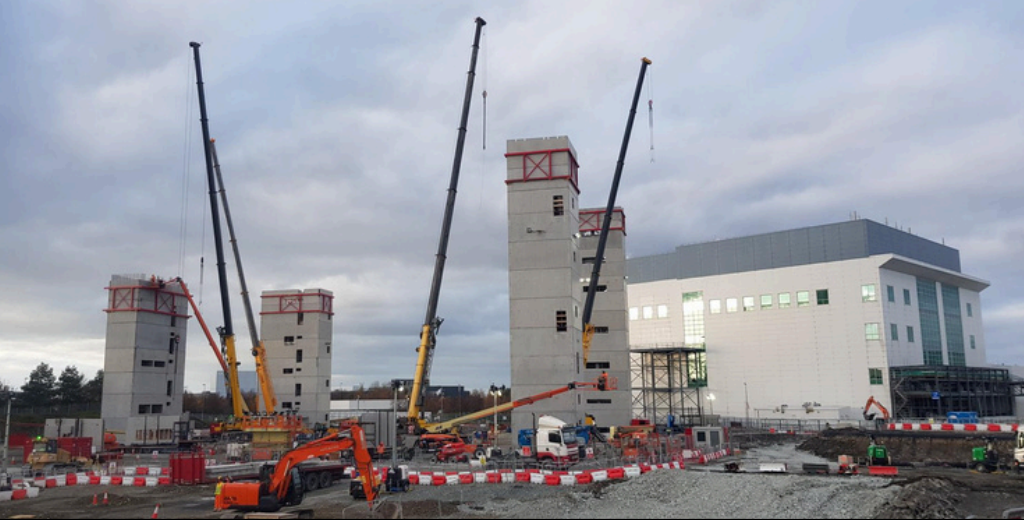
Provided Cranes and lifting solutions to assist Tusker contracts in erection of 8 no. Precast cores
